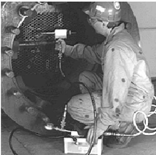
Figure 312-4.2-3 Typical Installation of Mechanical Fit Tube Plugs
